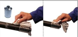
Remove emery cloth remnants with a clean cloth. Clean the cable jacket and the connector in the intended area with solvent cleanser e.g. with cable cleaner (e.g. CA-CLEAN-500), alcohol or spirit.
